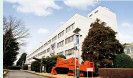
Tsuchiura Works East Building and the Hitachi UH03 hydraulic excavator, which is included in the list of Japan's Mechanical Engineering Heritage.
