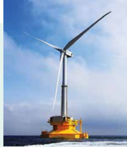
A 5 MW floating wind turbine (courtesy of the Fukushima Offshore Wind Consortium).
