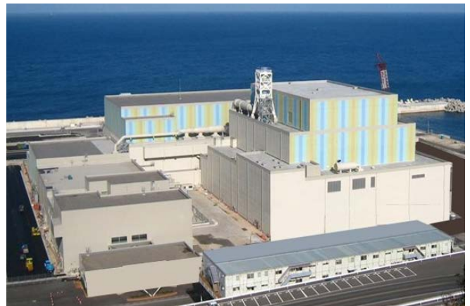
The Chugoku Electric Power Co., Inc., Shimane Nuclear Power Station Unit 3 (under construction)
