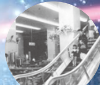
1949 Development of urban infrastructure
