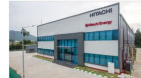
New valve and C&P 1 factory: Chennai, India
