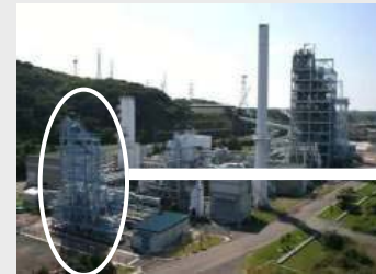
EAGLE pilot plant
