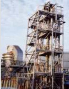
Pilot test (To 1995) Joint research by power companies
