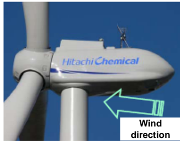
1st commercial unit (Completed Feb. 2008)
