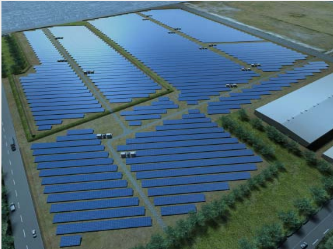
13MW-class Mega-Solar System for TEPCO, Ohgishima (Feb. 2011)
