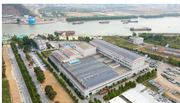
Photovoltaic installation, Zhongshan, China
