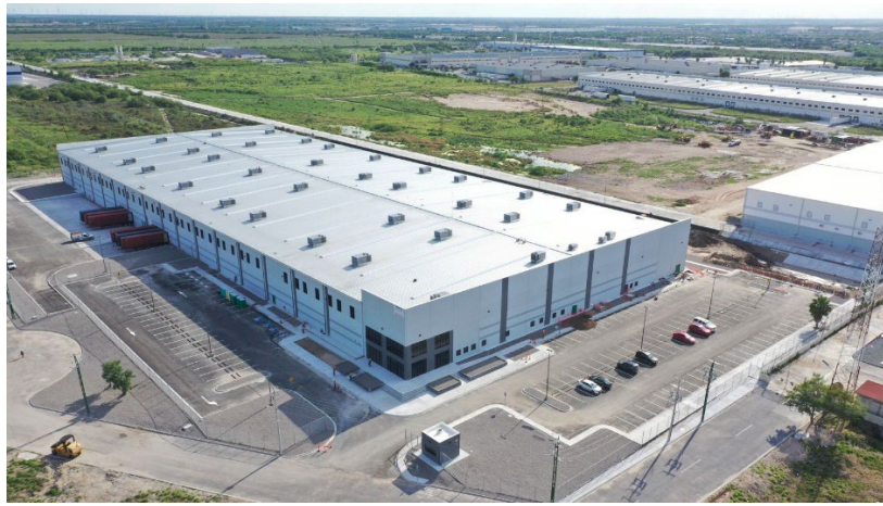
Hitachi Energy distribution transformer factory in Reynosa, Mexico
