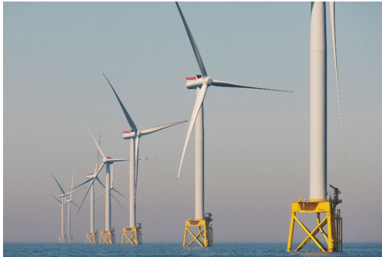
East Anglia One offshore wind farm. Courtesy of ScottishPower Renewables
