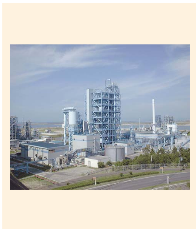
View of EAGLE pilot plant
