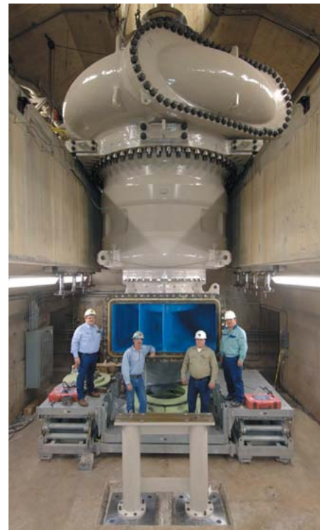
Completion of pump assembly
