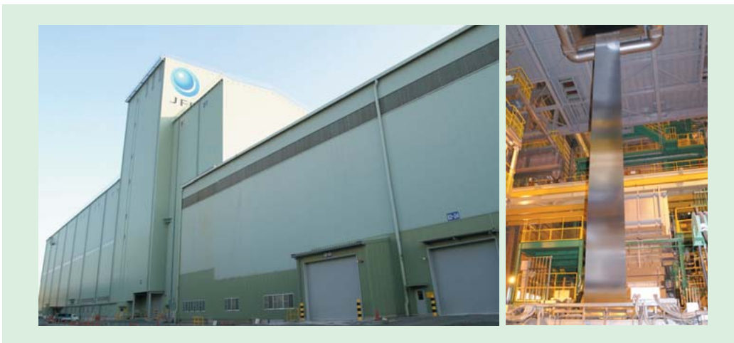
Outside view of West Japan Works of JFE Steel Corporation (left) and galvanizing equipment department (right)
