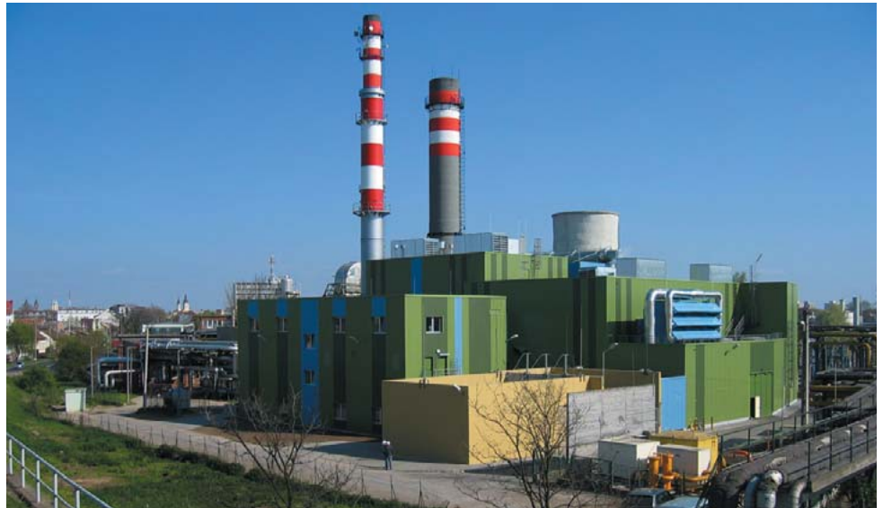
Full view of buildings making up the power generation facilities of E.ON Hungaria
