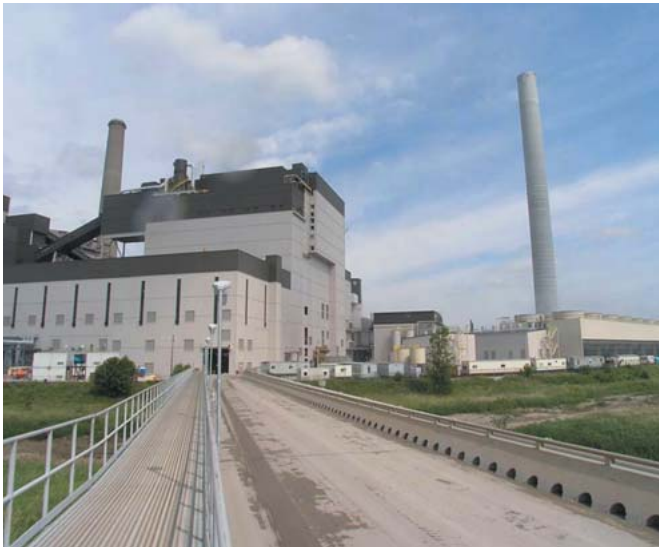
Building housing for steam turbines and boilers for MidAmerican Energy Company in USA
