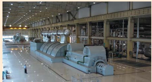
Appearance of the Zouxian Power Plant fourth phase (upper) and turbine-generators (lower) (foreground: No. 7 plant, background: No. 8 plant) in Shandong, China
