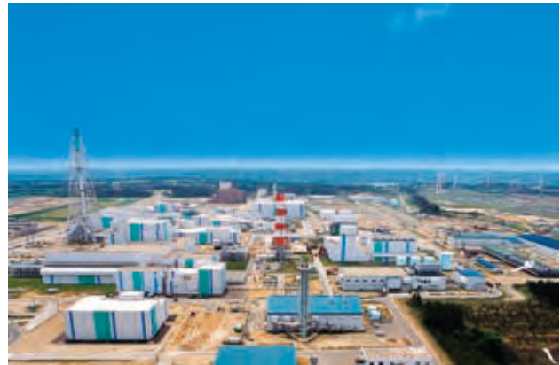
Fig. 3—Rokkasho Reprocessing Plant. View of the Rokkasho Reprocessing Plant site (photograph courtesy of Japan Nuclear Fuel Limited). The plant has a maximum annual reprocessing capacity of 800 tU and utilizes technology from France, the UK, Germany, and Japan.
