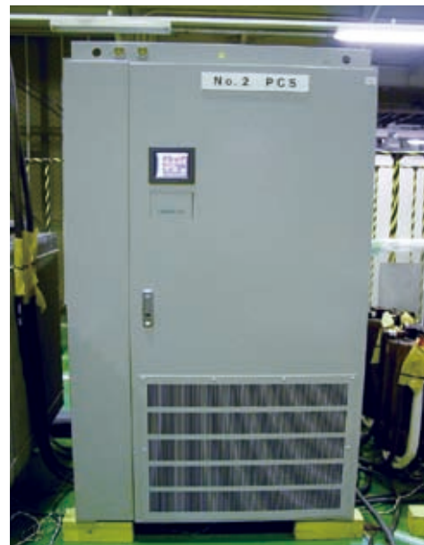
Fig. 3—PCS for Mega-solar. A large-capacity PCS (400 kW, 420 V, 3 phase) for large solar power generation systems (“mega-solar”).
