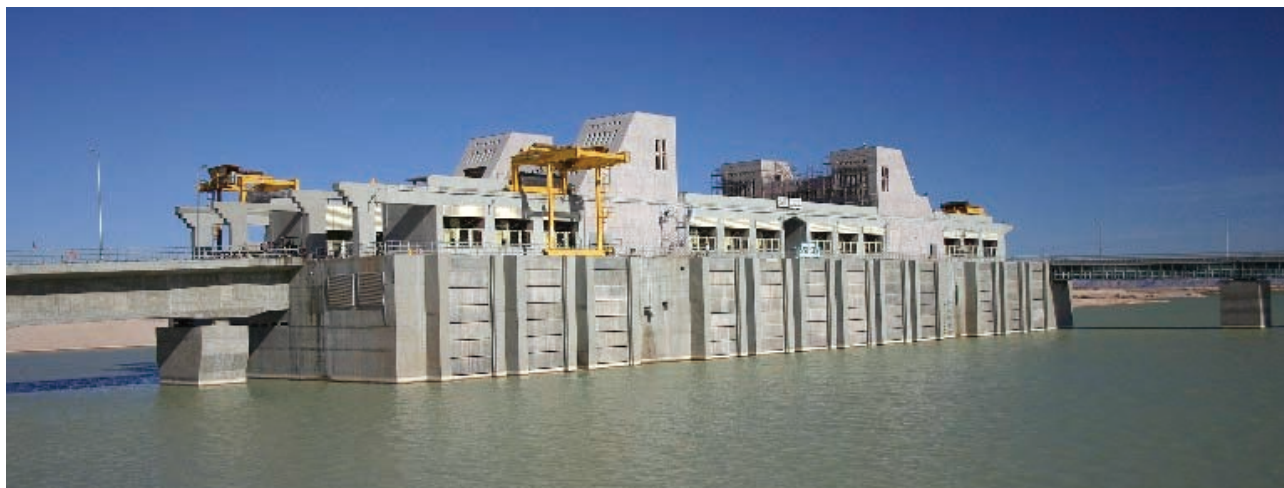
Fig. 2—Mubarak Pumping Station.
