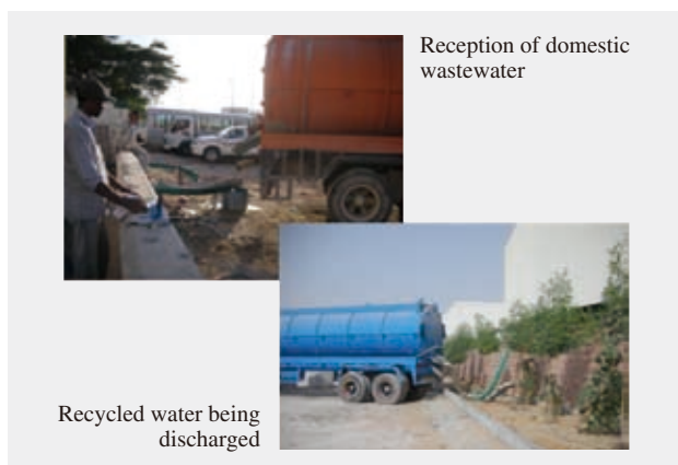
Fig. 4—Operation of Water Recycling Business in Dubai. Domestic wastewater is delivered by wastewater tanker for processing using MBR (membrane bio-reactor) and RO (reverse osmosis) and the recycled water is transported for sale by a recycled water tanker.
