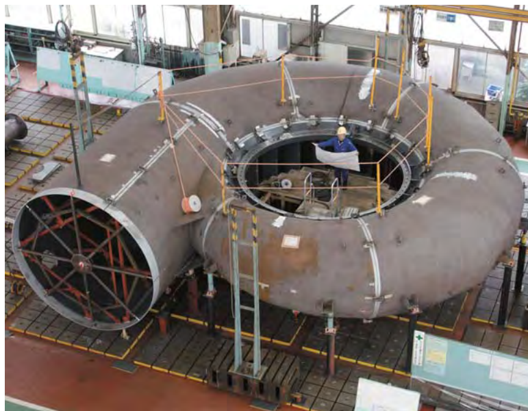
Turbine casing being assembled at factory
