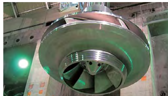
Installation of pump-turbine runner at Omarugawa Power Plant
