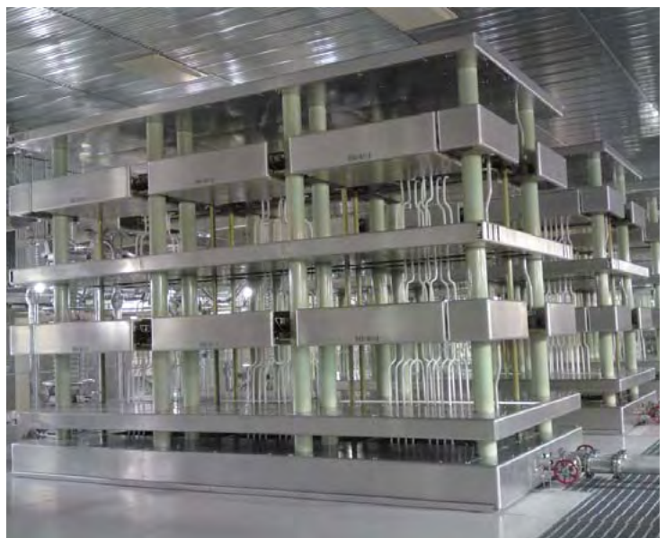
60-Hz-side thyristor valves for No. 1 FC
