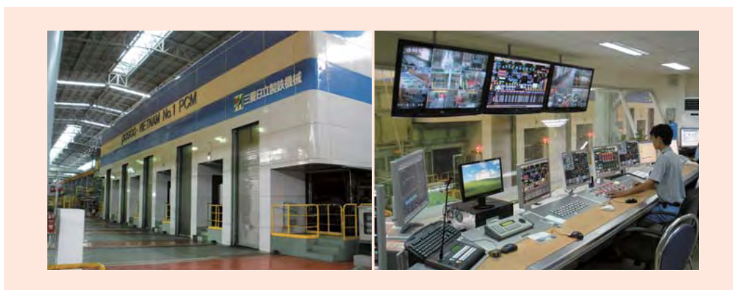
V1C continuous pickling line and cold rolling mill (left) and control room (right)
