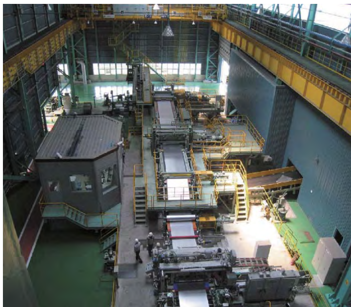
5CGL at Union Steel (entry side)
