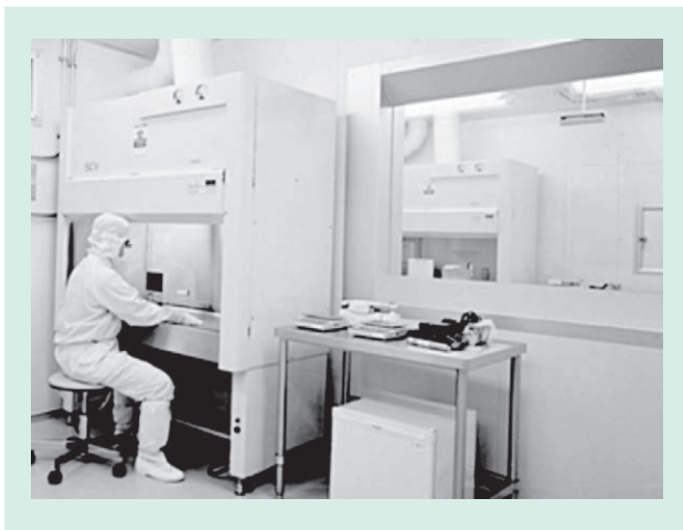
Fig. 4—CPF Interior. This scene from the Yotsugi CPF of the Donated Blood Distribution Foundation shows preparation work, which is performed in a safety cabinet in an environment-controlled room with 10 or fewer airborne microbes per cubic meter.
