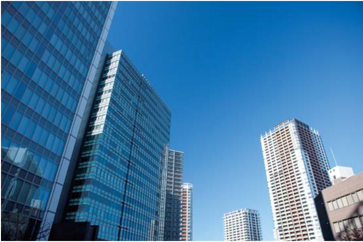
Service solutions for utility equipment
