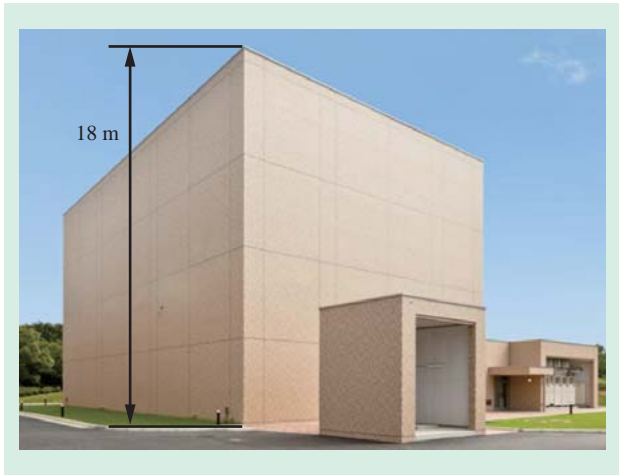
Fig. 7—Purpose-built Electron Microscope Building Providing Stable, Low-noise Environment.
