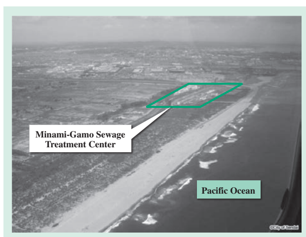
Fig. 1—Aerial View of Minami-Gamo Sewage Treatment Center. The Minami-Gamo Sewage Treatment Center, shown here after the earthquake, is located on the Pacific coast. Among the damage caused by the tsunami was the washing away of the coastal forest.
