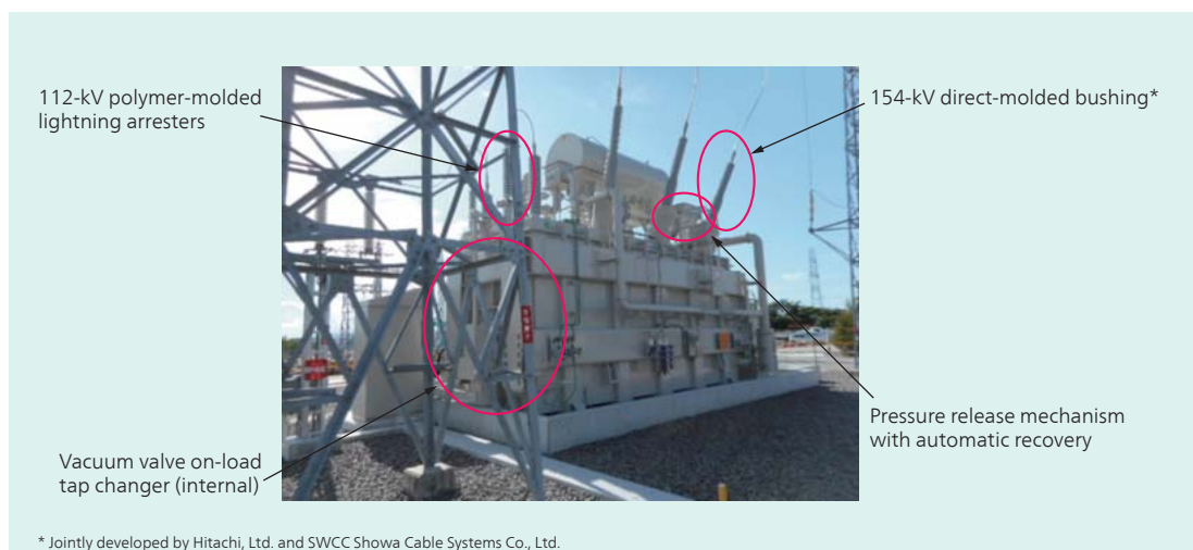
9 154-kV-class earthquake-resistant transformer for Tohoku Electric Power Co., Inc.
