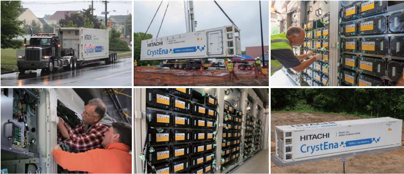
On-site installation at project in New Jersey, USA
