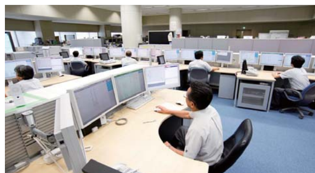
8 Tokyo region equipment command system (control system)
