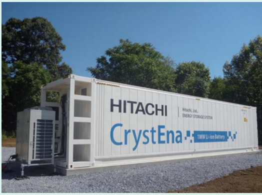
8 1-MW container-type energy storage system for ancillary services (left) and 500-kW power conditioner (right)
