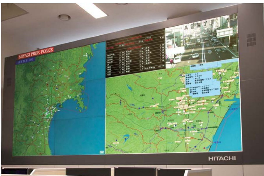
9 Large display for communication and command system for Miyagi Prefectural Police Headquarters
