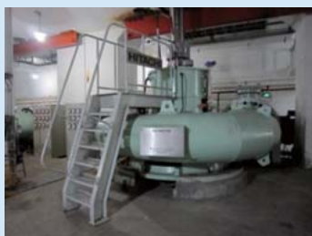
25 Specifications (top) and exterior (bottom) of high-capacity pump for the large-scale Yellow River Water Conveyance Project (China)
