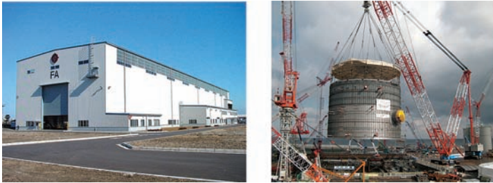
(Left) Module assembly factory (Hitachi Works, Hitachi GE Nuclear Energy)
