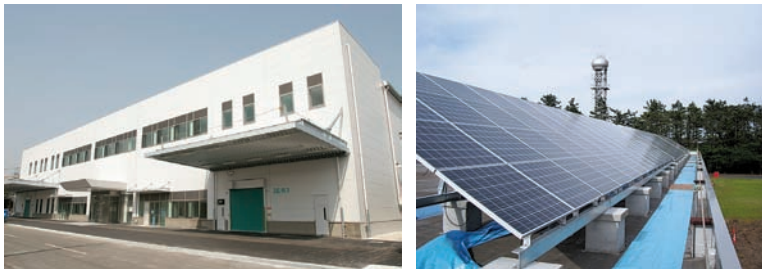
Narashino Division, Hitachi Industrial Equipment Systems Co., Ltd. (Right) The new production building uses high-insulation glass and energy-saving equipment (Left) Solar panels installed on the roof of the production building
