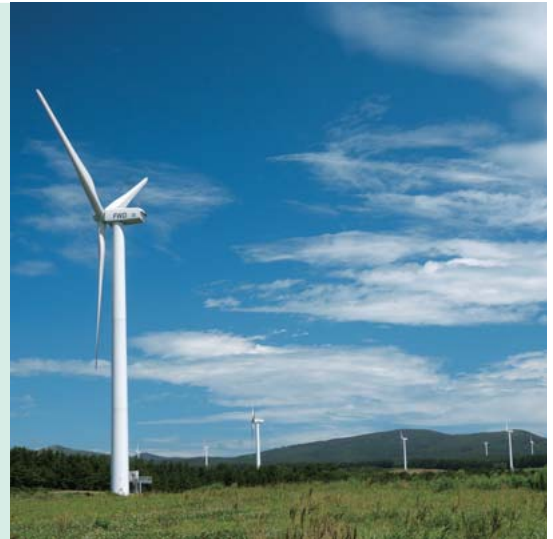
Rokkashomura-Futamata Wind Power Station
