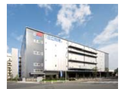
Hitachi Transport System's Keihin Distribution Center, a distribution center equipped with security systems
