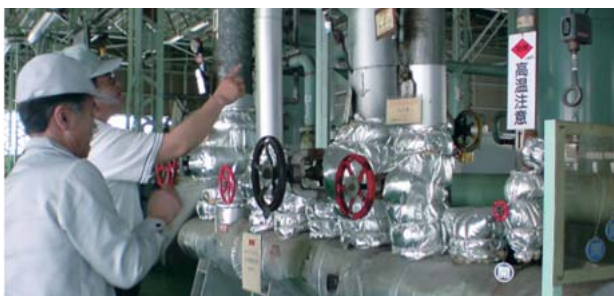
On-site energy conservation diagnosis
