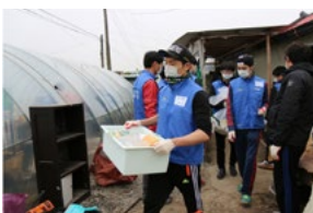
Volunteers of Kokusai Electric Korea repairing housing.
