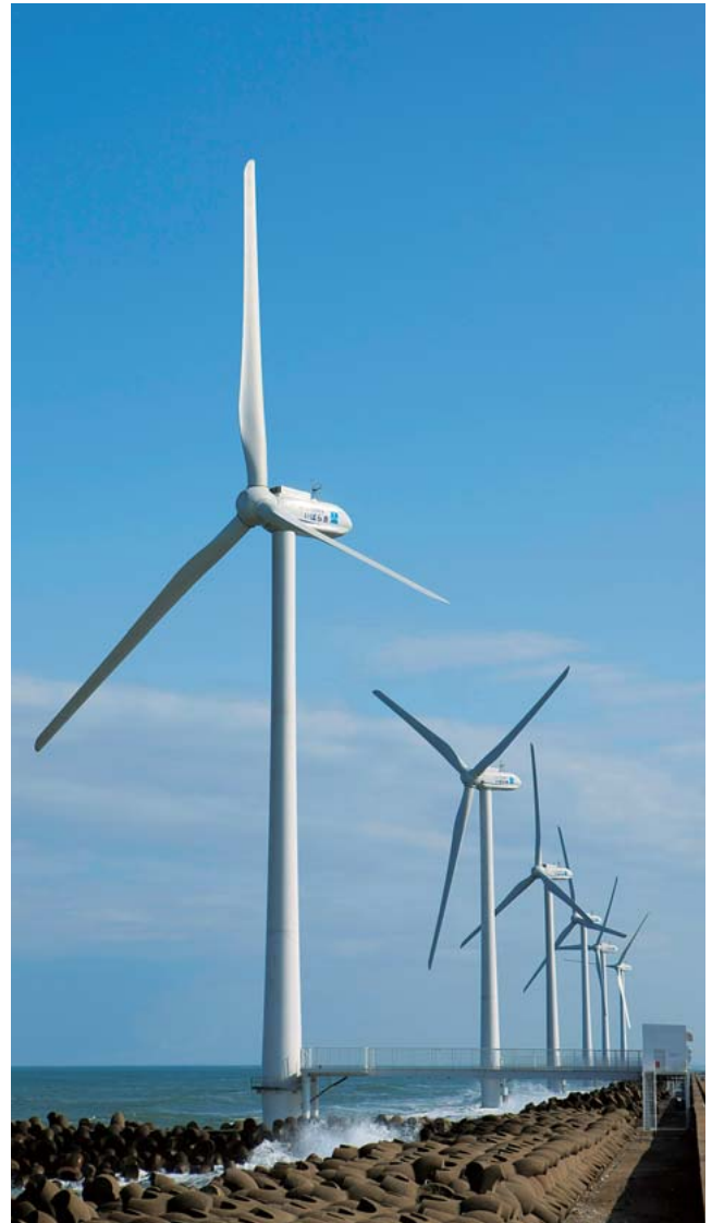
Wind Power Ibaraki Co., Ltd's Wind Power Kamisu
