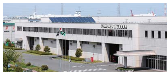
Solar power (maximum output 10 kW) is used at the plant
