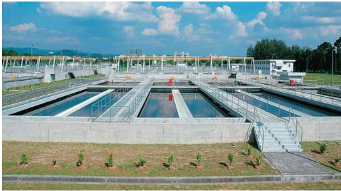
Bunus sewage treatment plant in Malaysia
